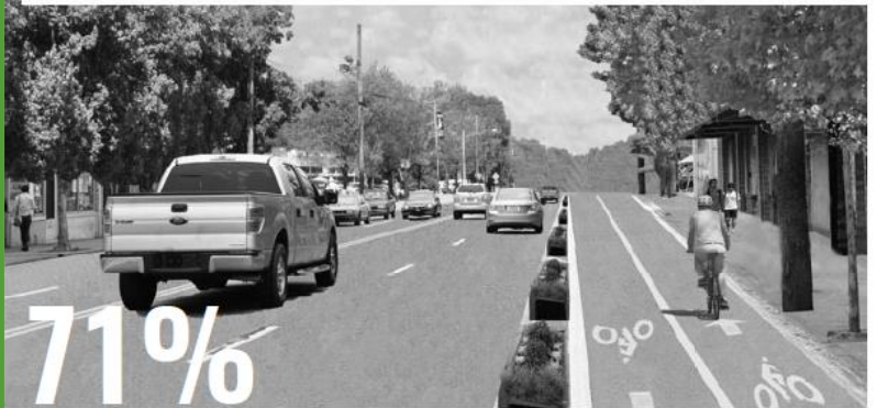
Bi-directional separated bike lane on a four-lane roadway.
