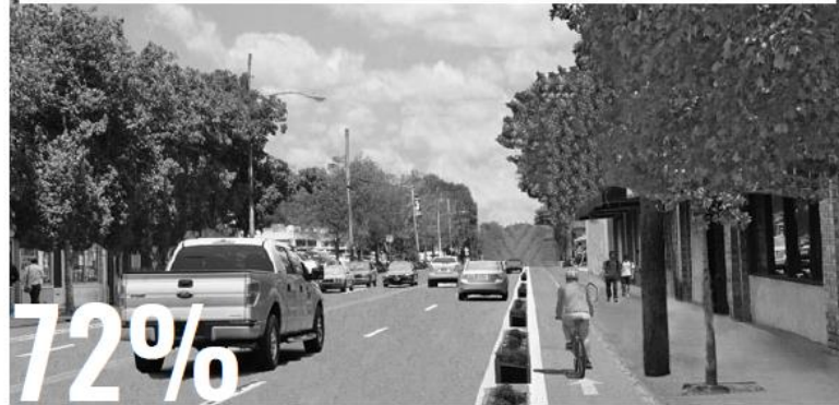
Separated bike lane on a four-lane roadway.
