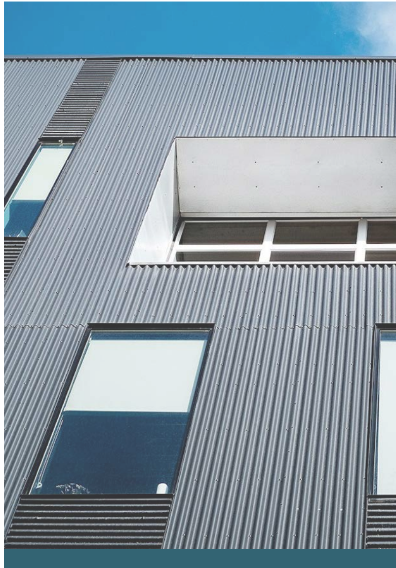
Building articulation through subtle changes in planes
